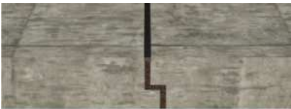
Discontinuous expansion joints
